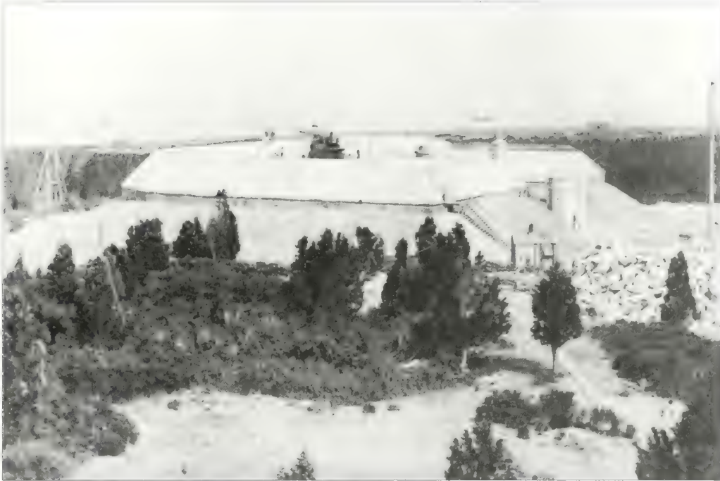
Figure 5.57. View looking southeast at Battery Potter, 1893. The Lift-Gun Battery #1, designated Battery Potter in 1903, was the only coastal defense battery constructed that used a steam-powered hydraulic lift to raise the guns up into firing position after they were loaded behind the protection of a massive concrete fortification (GATE 7811).
